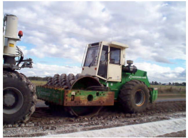
Figure 15 Padfoot roller following behind stabiliser
