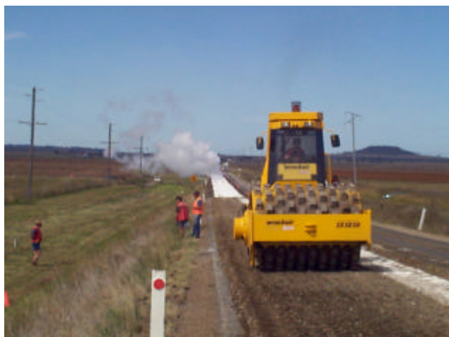
Figure 8 Slaking of quicklime and final compaction after stabilisation
