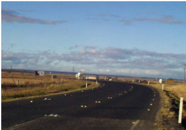
Figure 17 Sealed pavement at Nobby intersection
