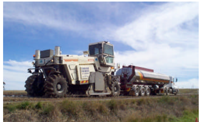
Figure 1 Insitu foamed bitumen stabilisation using Wirtgen WR2500
