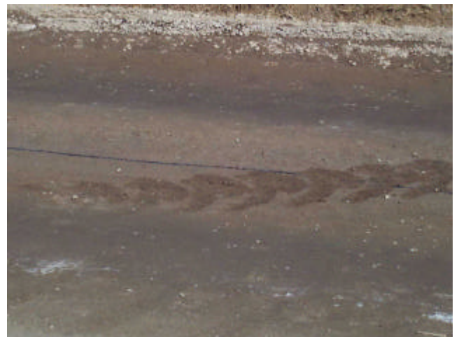
Figure 16 Foamed bitumen stabilised pavement after trafficking
