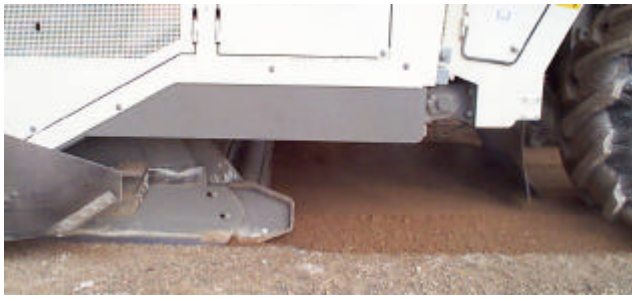
Figure 13 Freshly stabilised pavement material
