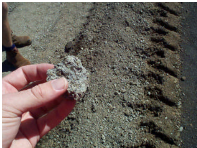
Figure 6 Pulverised cement treated patch
