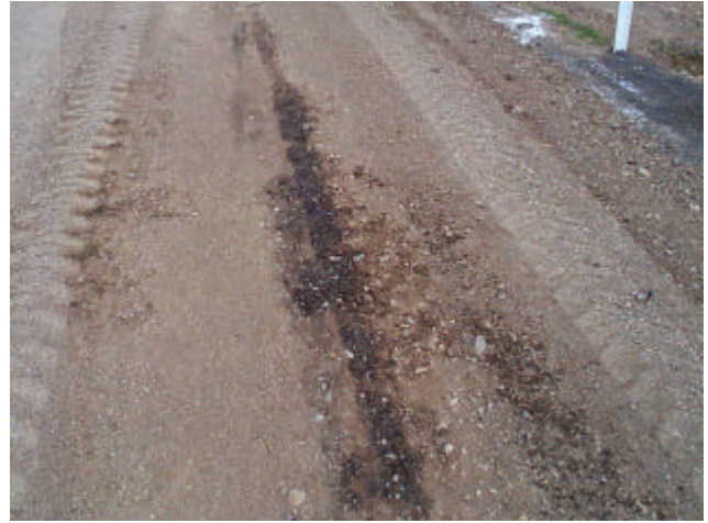
Figure 25 "Wet spot" over culvert
