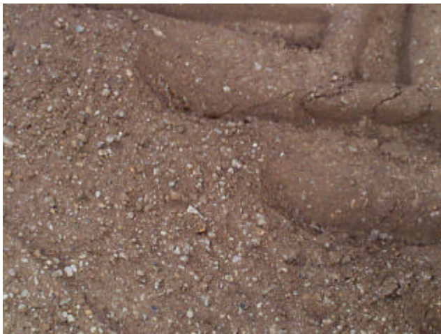
Figure 14 Freshly stabilised pavement
